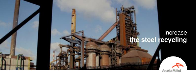
The project aims to increase the part of used steel (scrap) in the production process of the Fos-sur Mer steel mill. This involves adapting the scrap processing capabilities as well as installing an electric furnace (ladle furnace) downstream of the converter to compensate for the cooling of the liquid steel associated with this addition.
