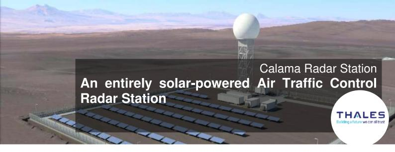
Thales is to deploy the world's first entirely solar-powered Air Traffic Control radar station in Calama, Chile. This system leverages 330 solar panels to take full advantage of the high levels of sunshine in the region. This solar radar station comprises an advanced primary radar and a secondary radar.
