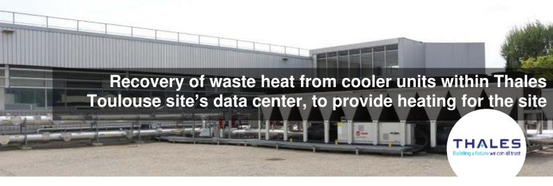
Thales has installed a heat recovery system within its data center on its Toulouse site in order to reduce its carbon footprint by replacing gas heating with a system that uses the calorific energy produced by the data center. It is also used for the cooling and air conditioning of less energy-consuming systems, adjusting when necessary for seasonal cold weather conditions.
