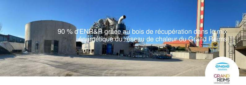
Grand Reims and ENGIE Solutions are working with the support of Ademe to integrate recovered wood ("bois B") into the energy mix of the Reims urban network. The development of this new energy source will produce 90% renewable heat by the end of the year. A two-year project that is fully in line with the achievement of the environmental objectives of Greater Reims: sustainably integrating the heating network into the urban fabric by promoting the use of renewable and recovered energy.
